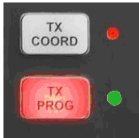
Detail of established connection in Prog Channel
